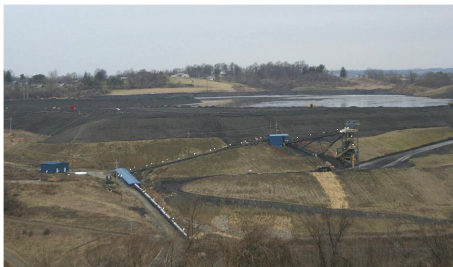
Far left: Mountaintop removal coal mine operation, Kayford Mountain, West Virginia. Above: A slurry pond; coal dust holding waste of coal mining. Photos by Creighton University student Ayet Nguyen. Courtesy of The Clifford M. Lewis, SJ Appalachian Institute. Top: http://www.wju.edu/ai/research/research.html#p=1
